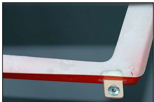
(below) Detail of the factory-finished canopy securing tongues, which are secured with M4 x 12mm bolts & T-nuts
