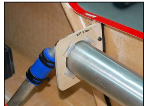
(below) Rear pipe mount is secured to a 3mm thick scrap plywood plate glued securely to the fuselage side.
